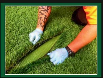
Fold back the turf on both sides of the seam, placing an object on the folded area if necessary to prevent it from unfolding. Position the seaming tape on the ground, securing its ends with stakes. Carefully remove the tape's protective layer and gradually join the two turf sections, ensuring alignment and preventing the blades or thatch from curling onto the tape. A zipper-like motion facilitates this step and is more efficiently accomplished with two individuals.
